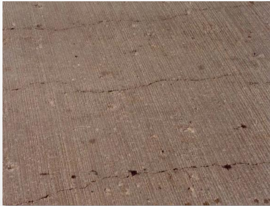
Cracking (shrinkage, ASR, loading)
