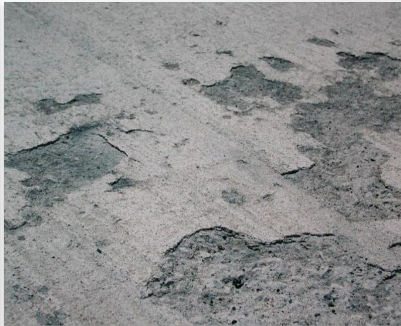
Spalling (freeze/thaw, carbonation, corrosion)
